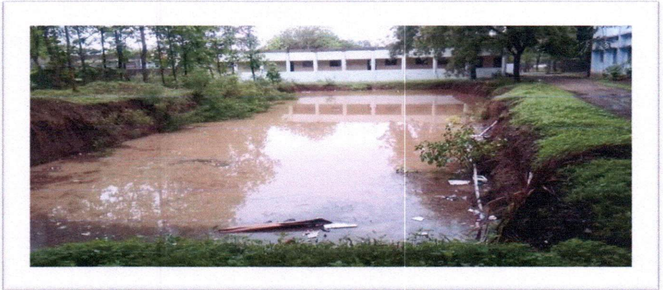
Check Dam Constructed in the campus
